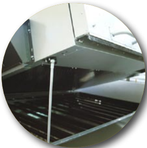
Outer cladding insulation layer
